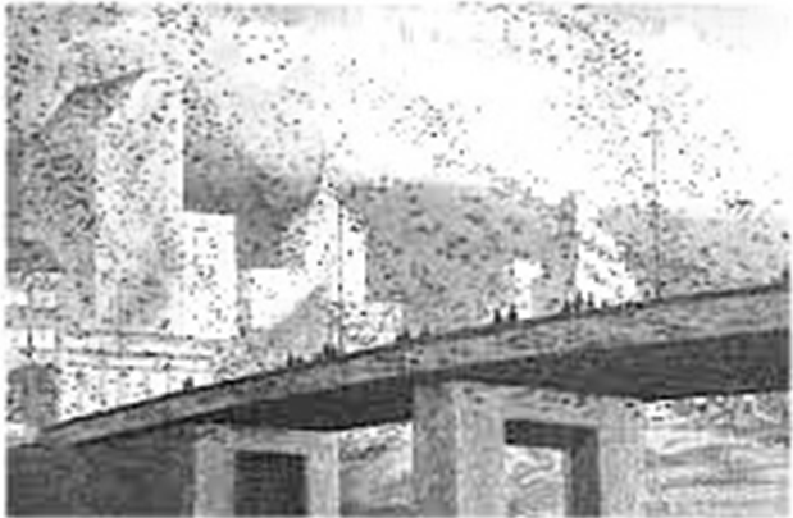
THE BRIDGE WITH BATS
