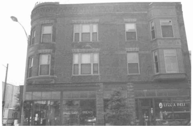
Looking at the north side of the Niles Building as it is today.
