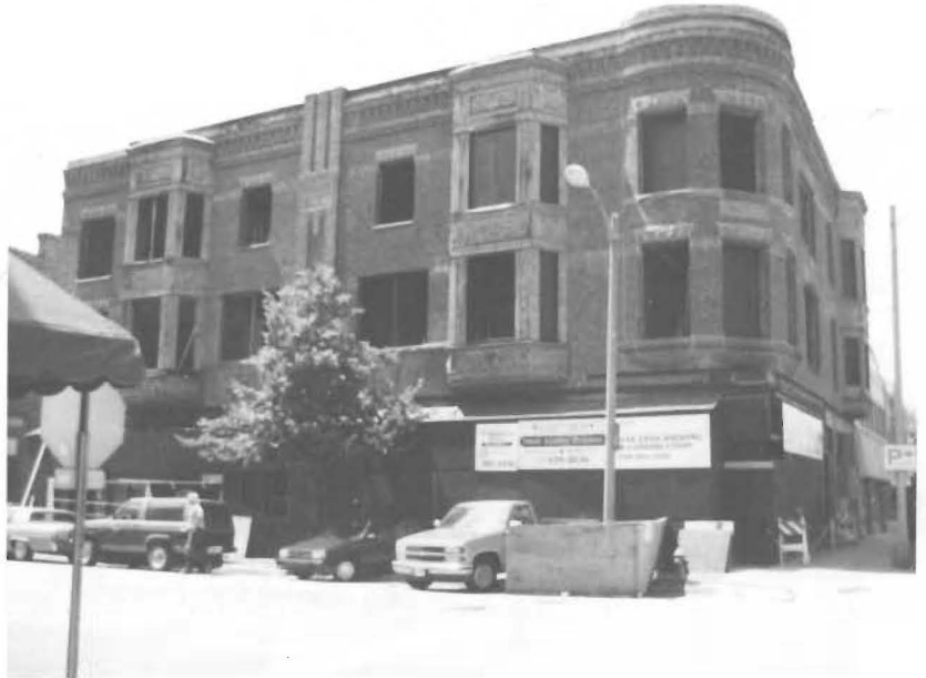
Above - The Niles Building being renovated in 1992.
