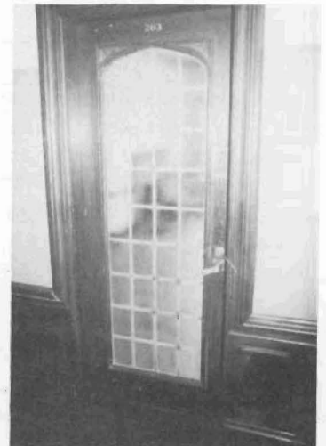
Doors throughout the building.
