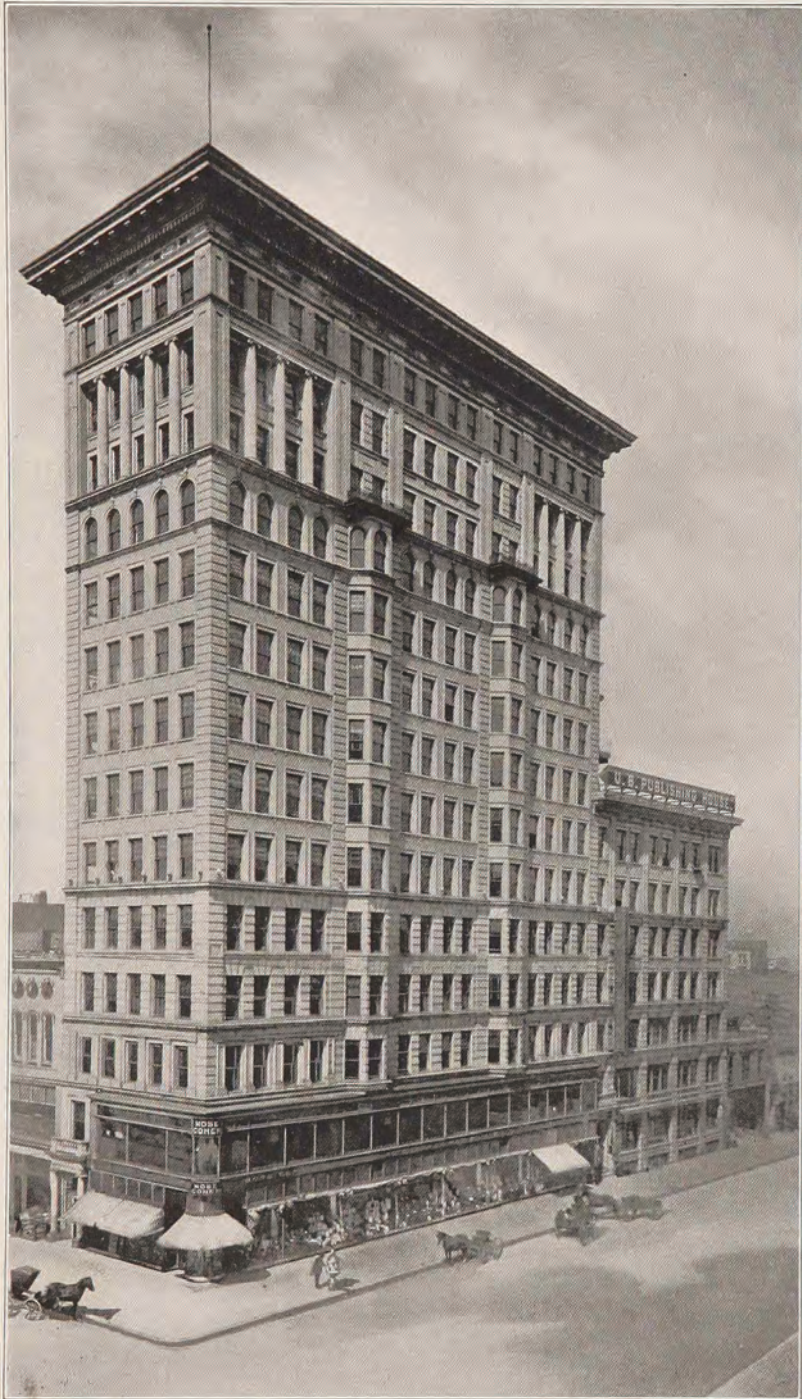
U. B. OFFICE BUILDING DAYTON, OHIO
